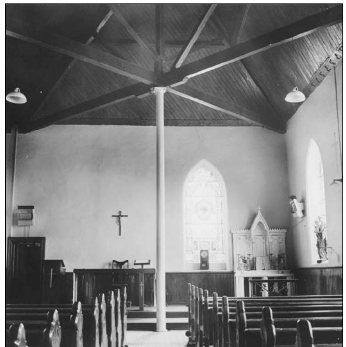
Photo 1: Looking up the interior of the Men's House, Keash R.C. Church, Co. Sligo, as it was prior to the start of renovations in 1977.
